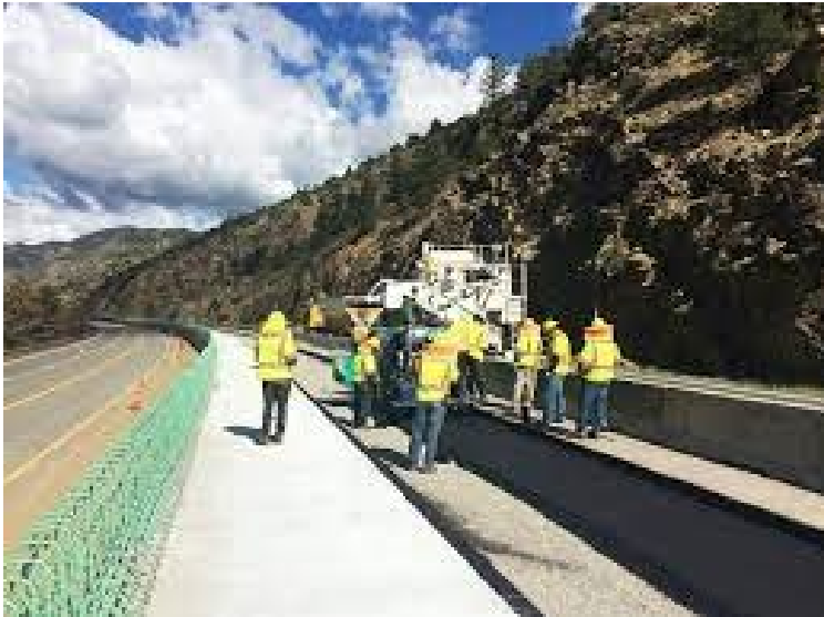
Westbound PPSL Construction
